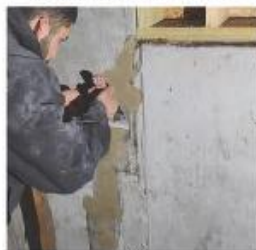
We patch with CONCRETE FUSION Crack Repair Product
