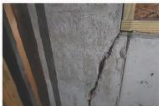
Foundation Crack
