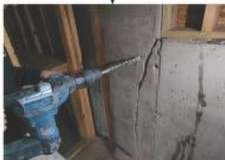
We drill holes for our Staple System
