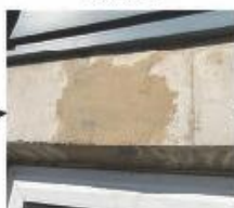
With CONCRETE FUSION Crack Repair Product
